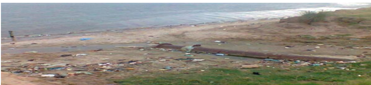
Fig 4: showing underground pipe run into the Lagoon in Lagos Metropolis
